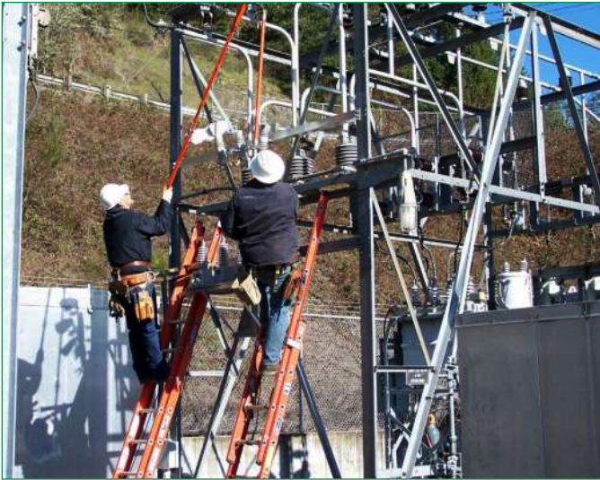
Lane County Co-Op
